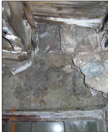
Ground floor stonework
