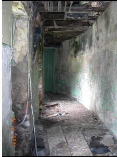
First floor of west range
