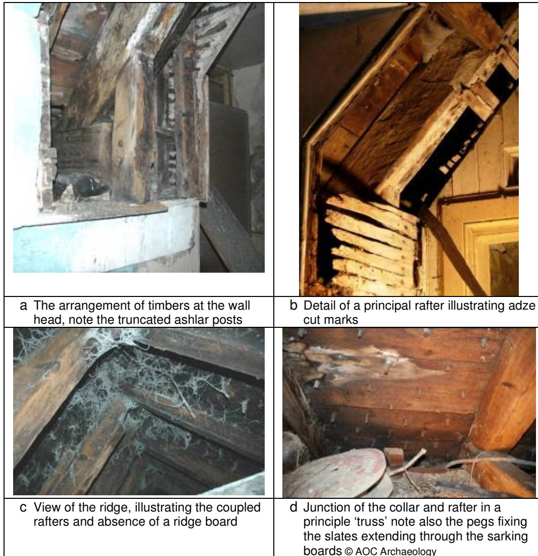
Figure 30: Details of the south range roof
