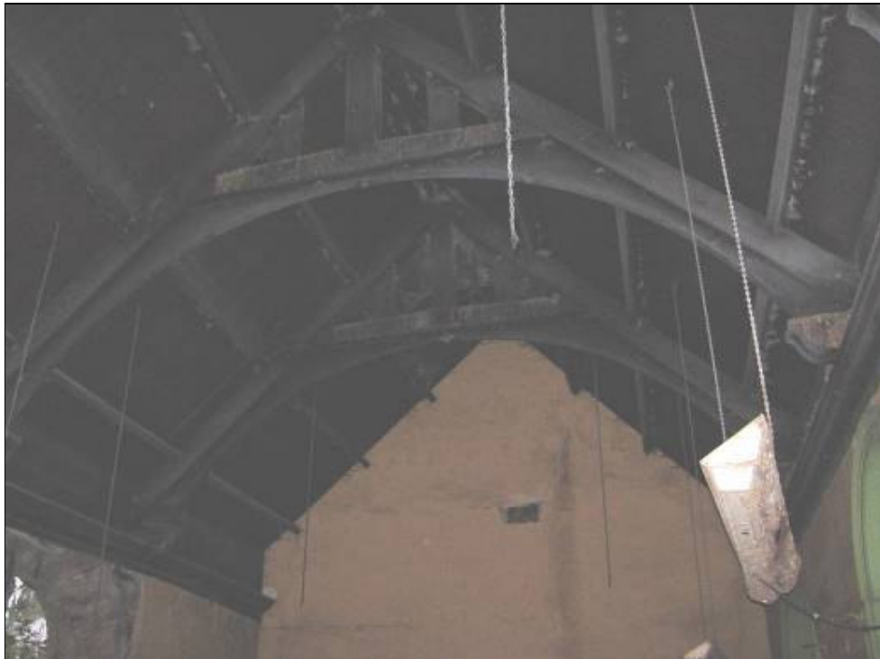
Figure 28: The roof structure over the main hall
