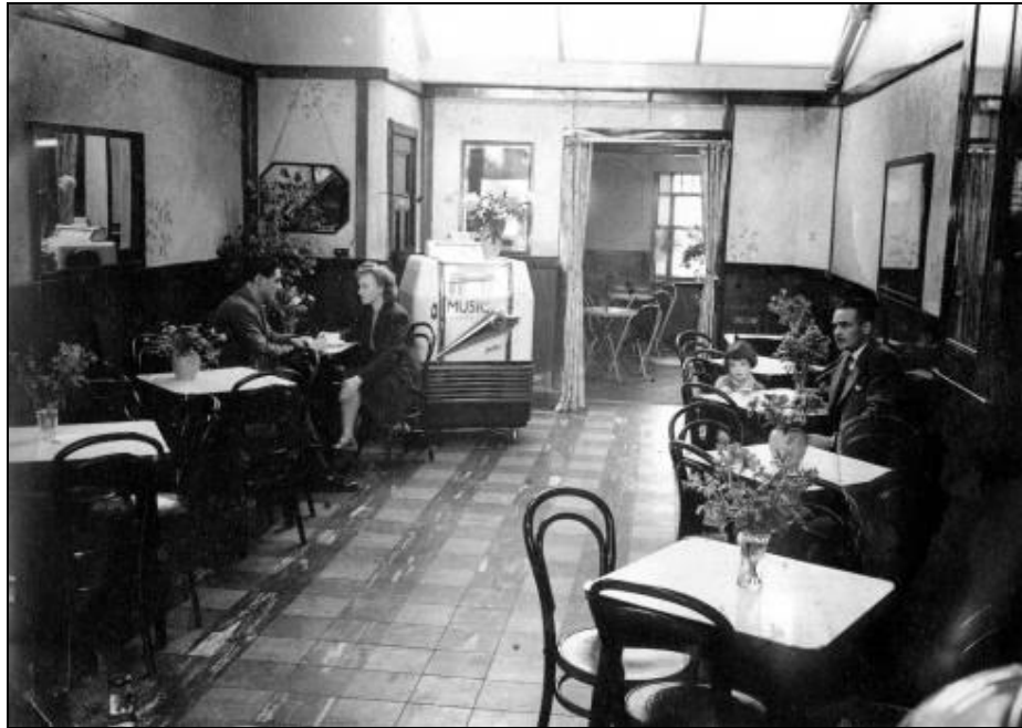
Figure 23: The Locarno Café looking north into the south range of the Old Courthouse
