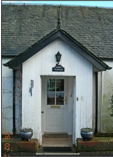
Figure 40: Traditional front porches to Tadmore and Murray House, note the modern pattern, uPVC and pressed steel door to Tadmore
